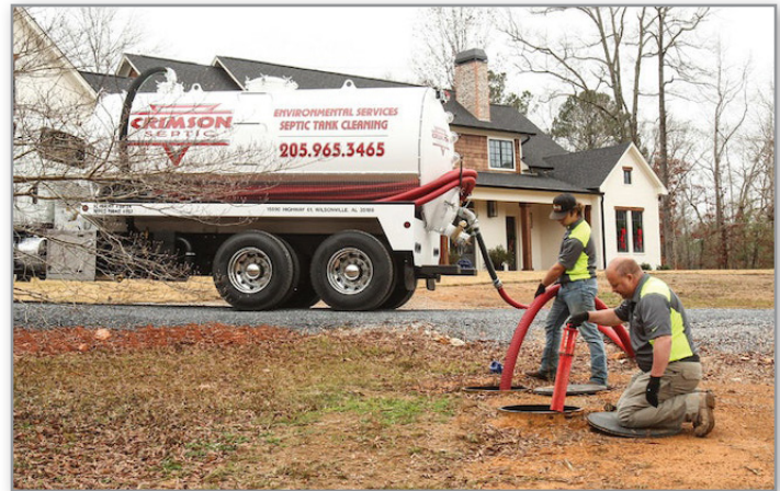
Shane Seale, in foreground, inspects an outlet filter as technician Logan Jackson pumps the inlet side of the septic tank.
